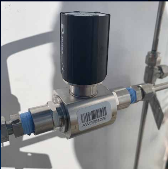
Differential Pressure Sensor ( Level Sensor)
